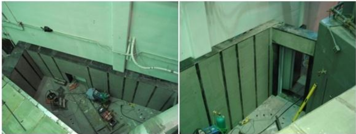
Fig. 2.33. Images of the assembly of the positron beam shielding cave.
